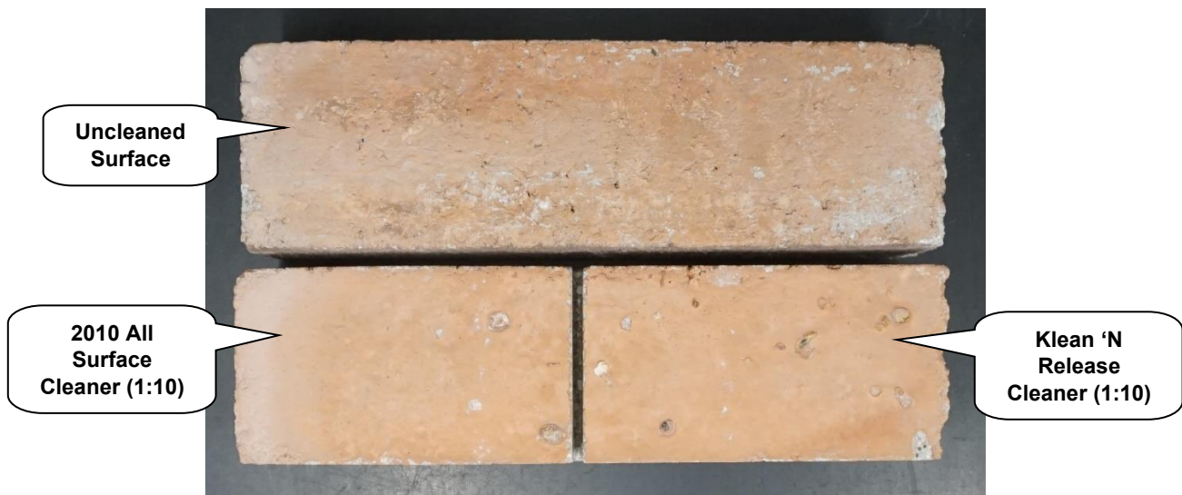
"Pinehurst" Concrete Brick After Cleaning
