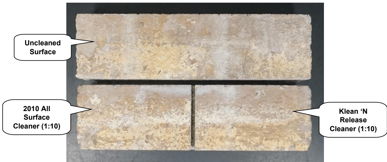
"Rhodes" Concrete Brick After Cleaning
