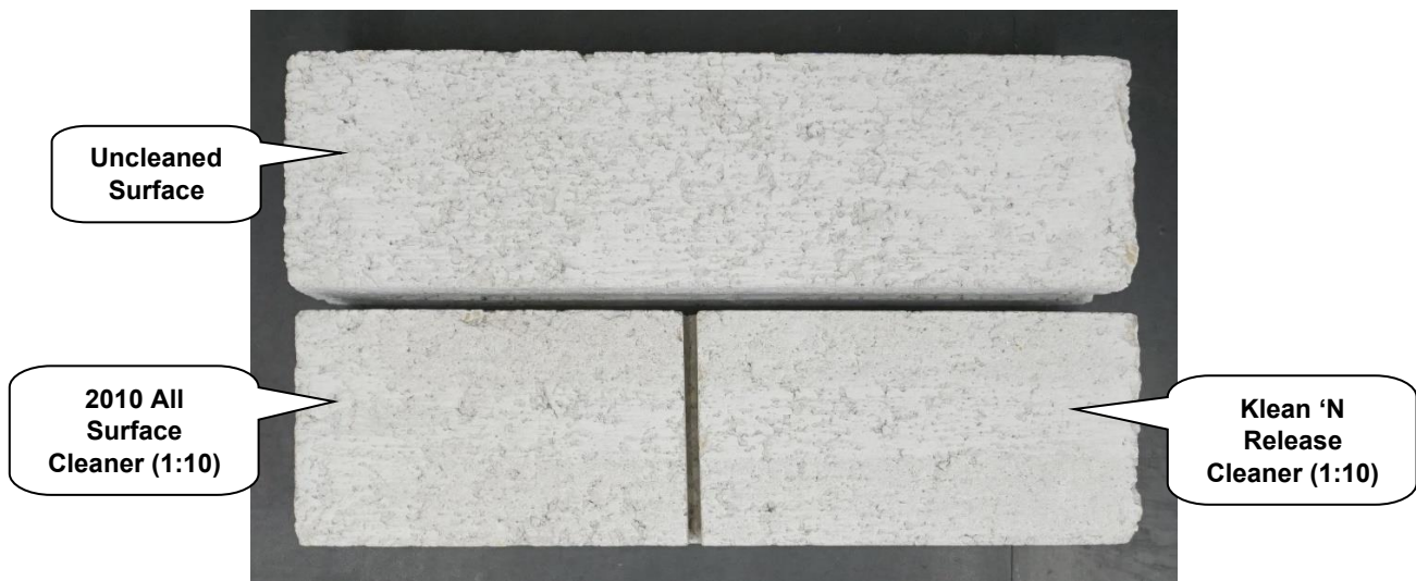
"Frost" Concrete Brick After Cleaning
